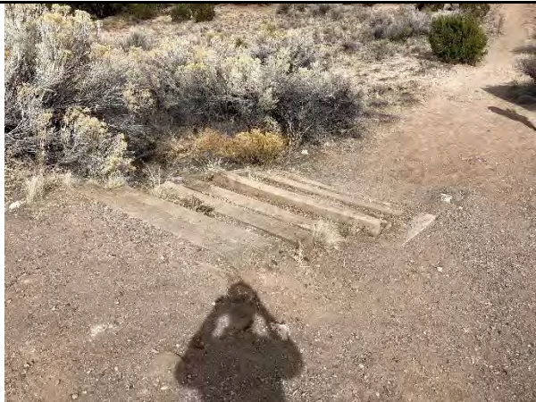
Existing stairs from street to trailhead
