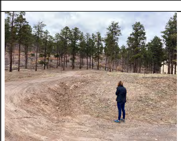
Access road/trail; lack of trail signage
