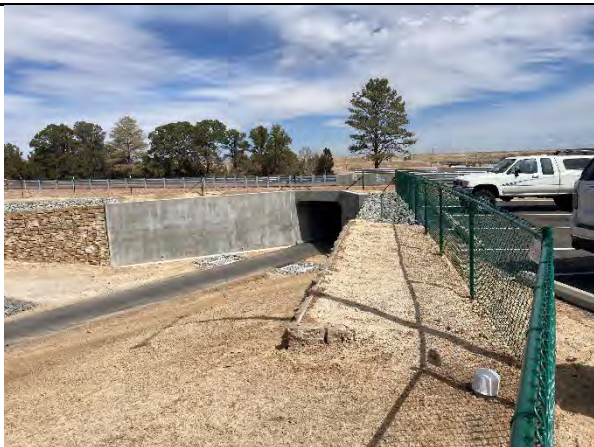
Below-grade connection across East Rd (502)
