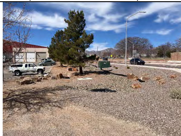
Unclear parking permission at Fire Station
