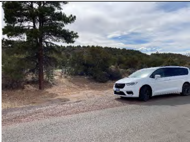
Steep embankment btwn St Rd 4 and access gate
