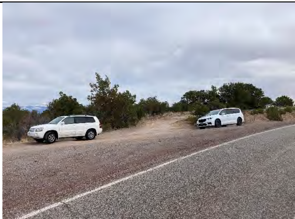
Pullout parking along State Road 4; ~ 3-4 cars
