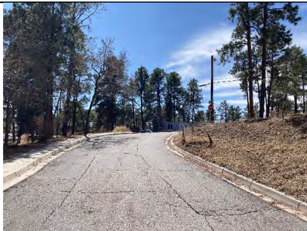
Access road looking up from tennis court
