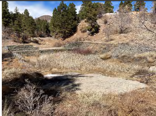
Drainage feature just beyond access point
