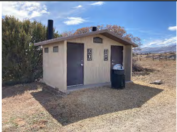
Restrooms further down trail at Brewer Arena
