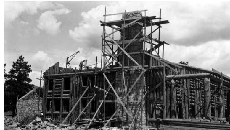
Lodge under construction, 1927.
